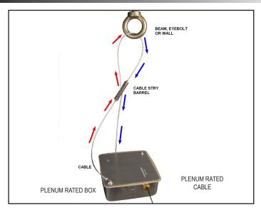
Wrap the cable around a beam, eyebolt or hanger. Next, slip the cable through the top of cable stay barrel pulling excess cable until taut.
