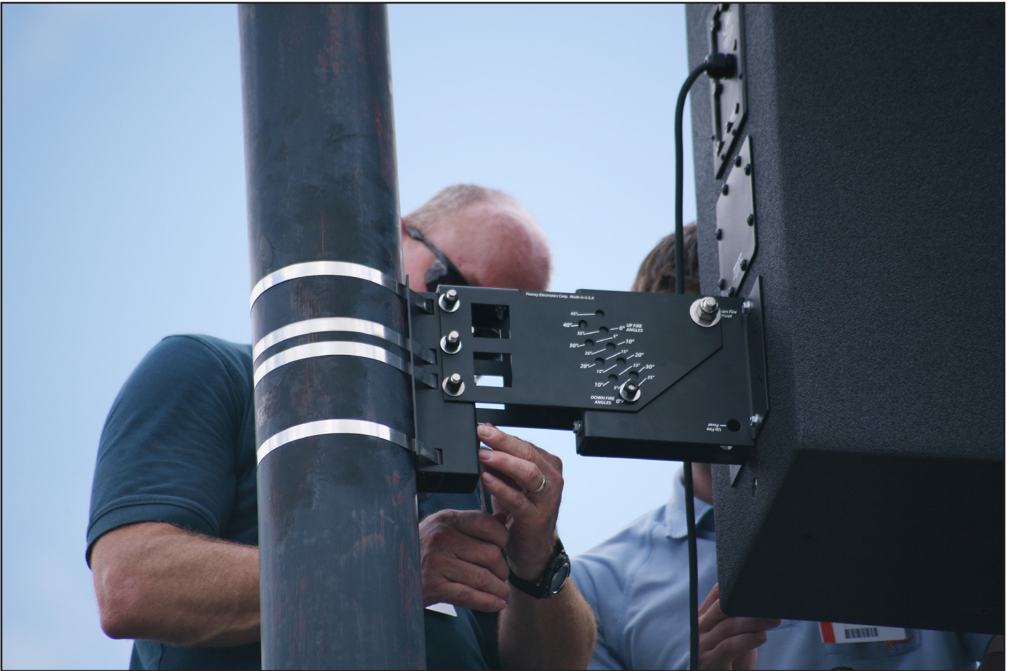
9. Secure pole mount to speaker mount using three bolts and nuts provided. (see picture above)
