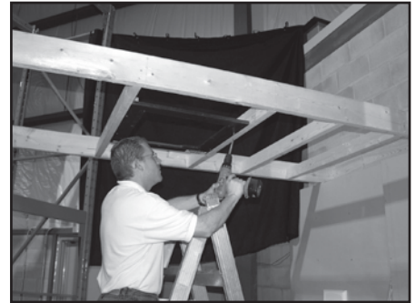
Fig. 3: Attaching pre-installation ring to blocking.
