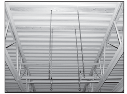
Fig. 13: Suspension points with turnbuckles installed.
