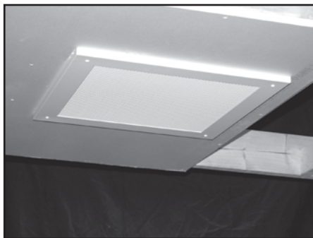
Fig. 10: Completed subwoofer installation.
