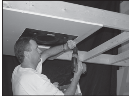
Fig. 8: Attaching the subwoofer to the pre-installation ring.
