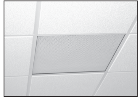
Fig. 10: Completed subwoofer installation.
