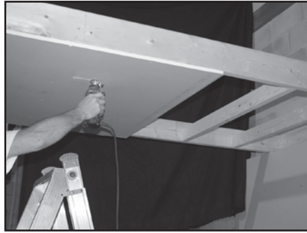
Fig. 5: Cutting drywall using the Rotozip™.
