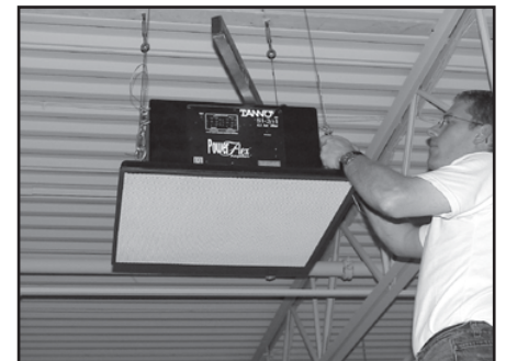
Fig. 16: Leveling the subwoofer.
